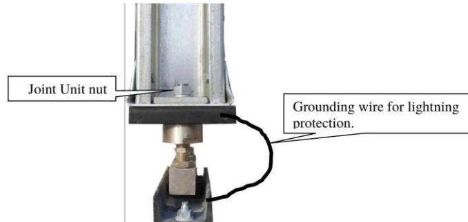
Drawing 6 – Joint unit nut with grounding-wire connection
